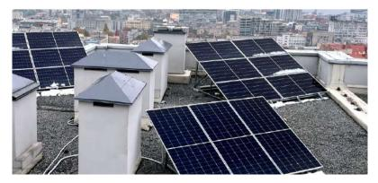
The HOA 'Geneva Dnipro' in the city of Dnipro has installed a 84.2 kW solar power station, a 96 kW inverter, and 102.4 kWh batteries thanks to the 'GreenDIM' Program. This has ensured uninterrupted power supply for the building's critical systems, including elevators, video surveillance, pump group, and lighting.
